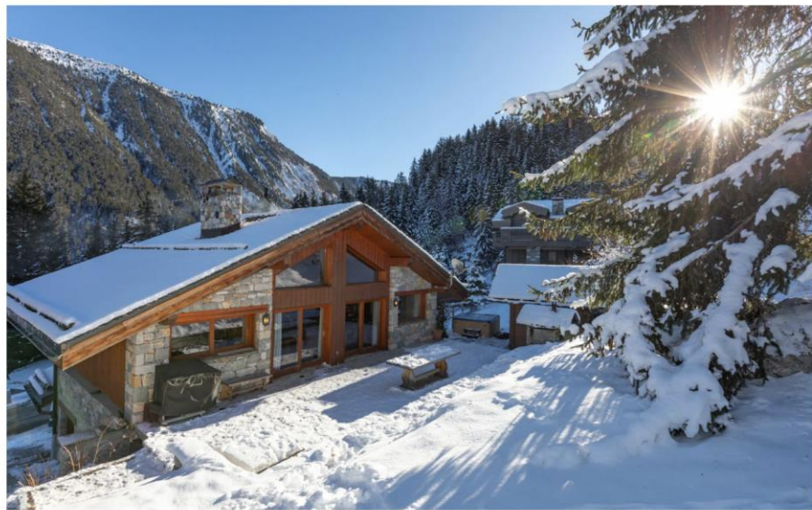
Chalet Rikiki in Courchevel has room for 22 people
